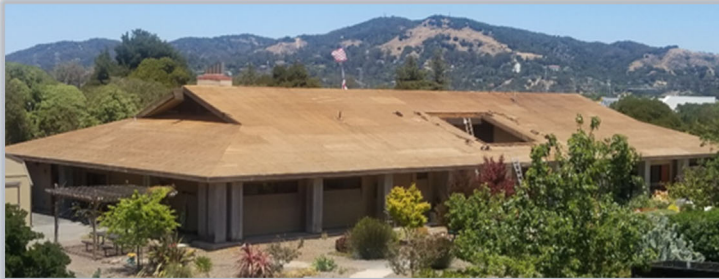
Demolition of old roof.
